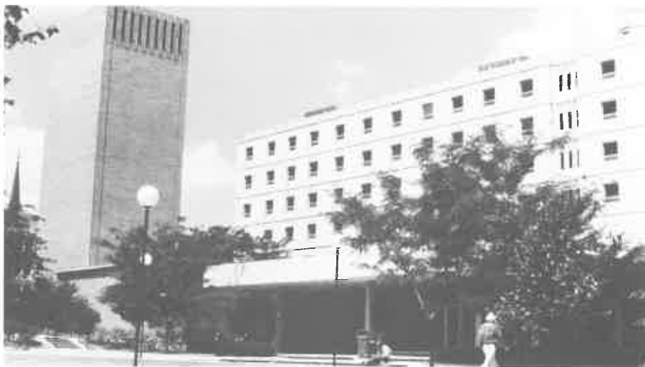
Van Allen Hall from the southeast
